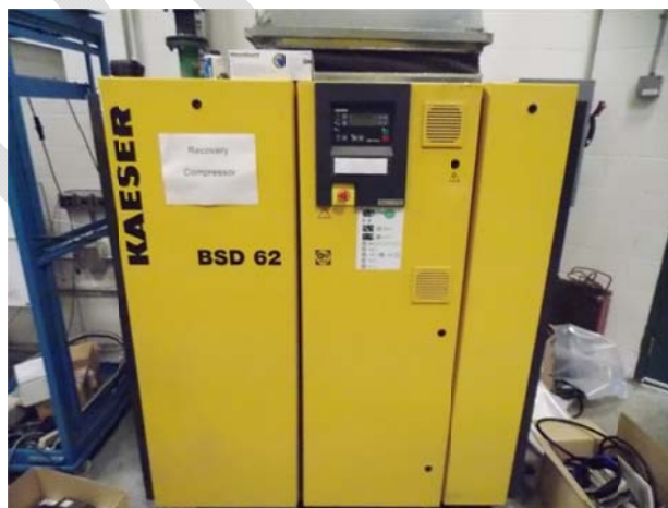
Figure 4.9.2.1.b – Helium recovery compressor (ISAC-II Helium Compressor Room 166).
