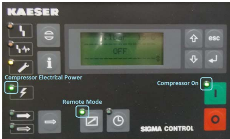
Figure 4.9.2.8.c – Helium recovery compressor panel; circled LEDs must be lit to enable startup.
