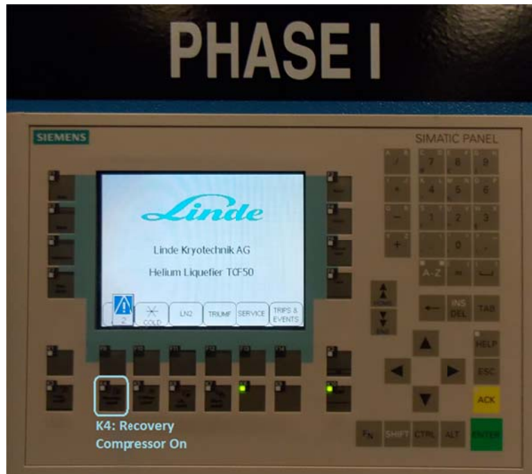
Figure 4.9.2.8.e – Phase-I Linde PLC control panel.
