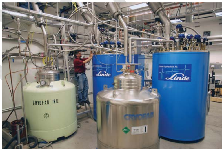
Figure 4.9.1.b –LHe supply dewars (foreground), Cold Boxes (blue, background); ISAC-II Cryogenics Room 164
