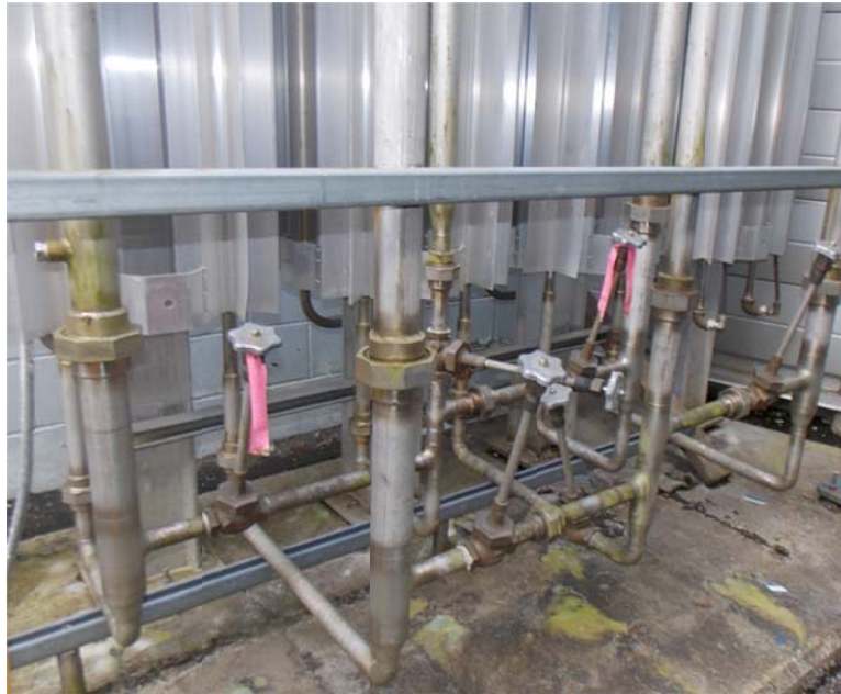
Figure 4.9.2.1.a – Ambient heat exchangers in the alleyway between ISAC buildings.
