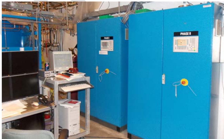
Figure 4.9.2.8.d –Phase-I (left), Phase-II Linde PLC control cabinets, ISAC-II Cryogenics Room 164.
