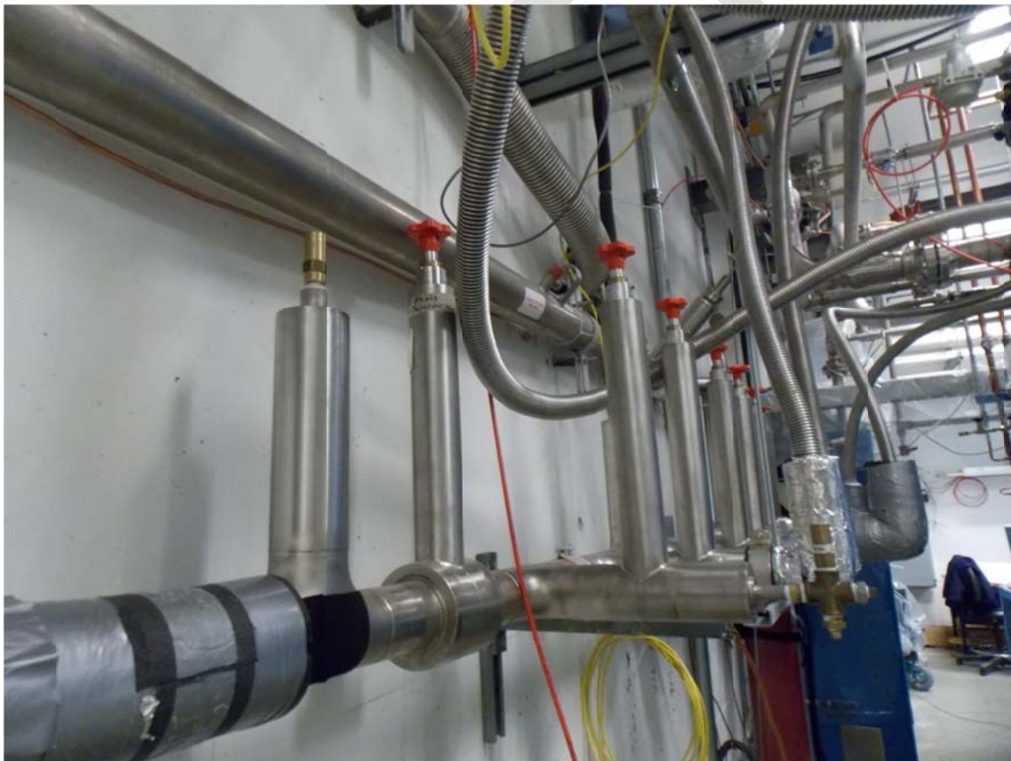
Phase Separator Nitrogen Supply valve (first red-topped valve on the left)
