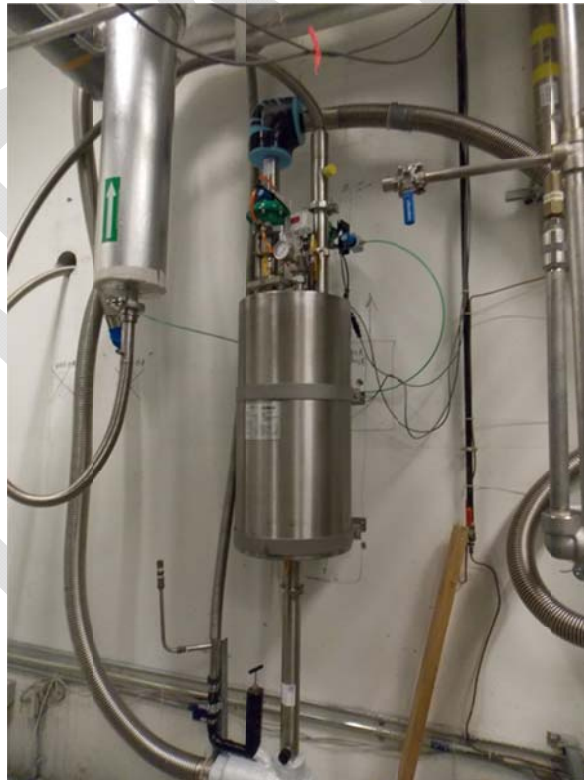
Figure 4.9.1.c – LN2 Phase Separator, ISAC-II Cryogenics Room 164, Northwest corner
