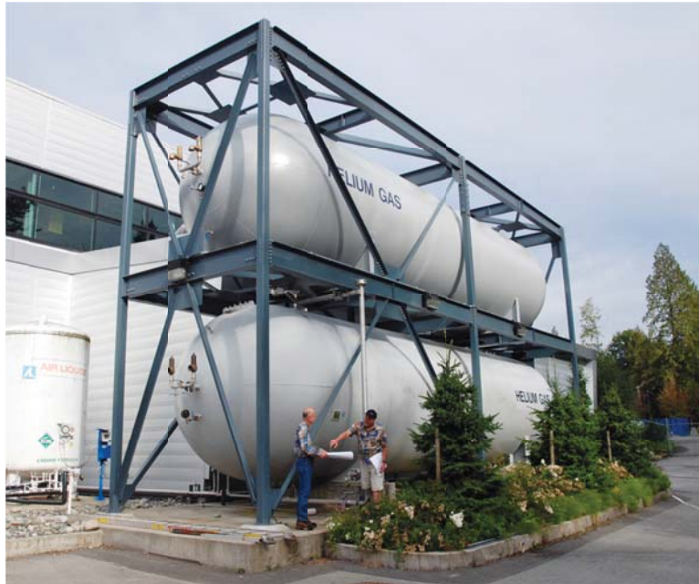
Figure 4.9.1.a – Helium buffer tanks, east of ISAC-II Experimental Hall.
